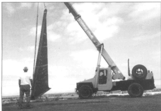
Fig 1: The gnomon in course of erection
